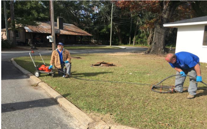
Tommy and Jimmy hard at work unstopping a sewer line at Cherokee Homes.
